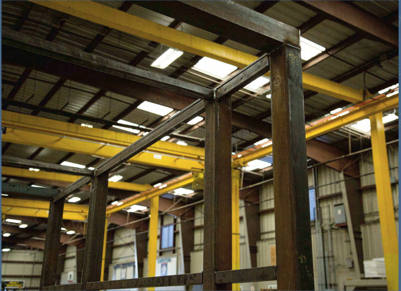
Steel framework for CALCTRA's concrete communication building
